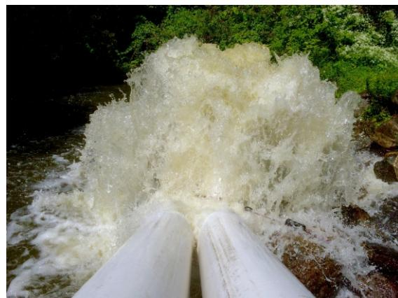
foot-long white tubes over the spillway and discharge ends shown in this photo to draw down the lake during the winter months. We do this every two to three years to cold shock and kill weed tubers.
