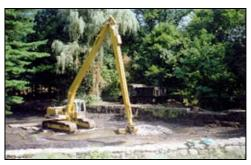
**Dredging:** This method is usually not solely used for aquatic plant control. Dredging is employed to deepen water that has been filled in from sedimentation (often sped up by man-made activities), remove excessive nutrients, or even remove toxic substances in the sediments. As a side benefit of these lake restoration projects, deeper water and nutrient removal often limits aquatic plant growth. Although long-term aquatic plant
