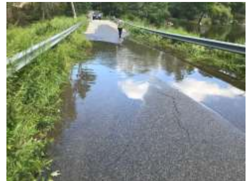
Our flooded bridge after IDA. The lake rose to 17" over the summer weir board!
